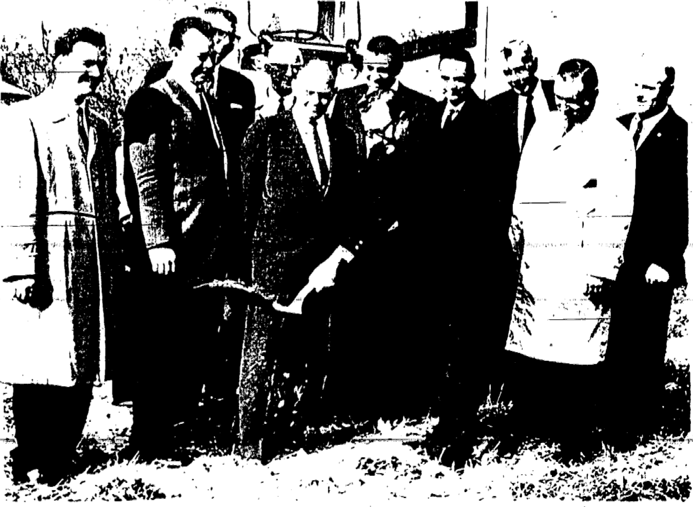
MAYOR FREDERICK WILHELM of Mountainside breaks ground for the borough branch of the First Federal Savings and Loan Association of Westfield. Taking part in the ceremonies, held last Tuesday at the Mountainide Inn, site of the new branch, are other borough notables including left to right, Councilman P. Wester, Councilman Raymond J. Herrcott, Borough Attorney Irvine B.
