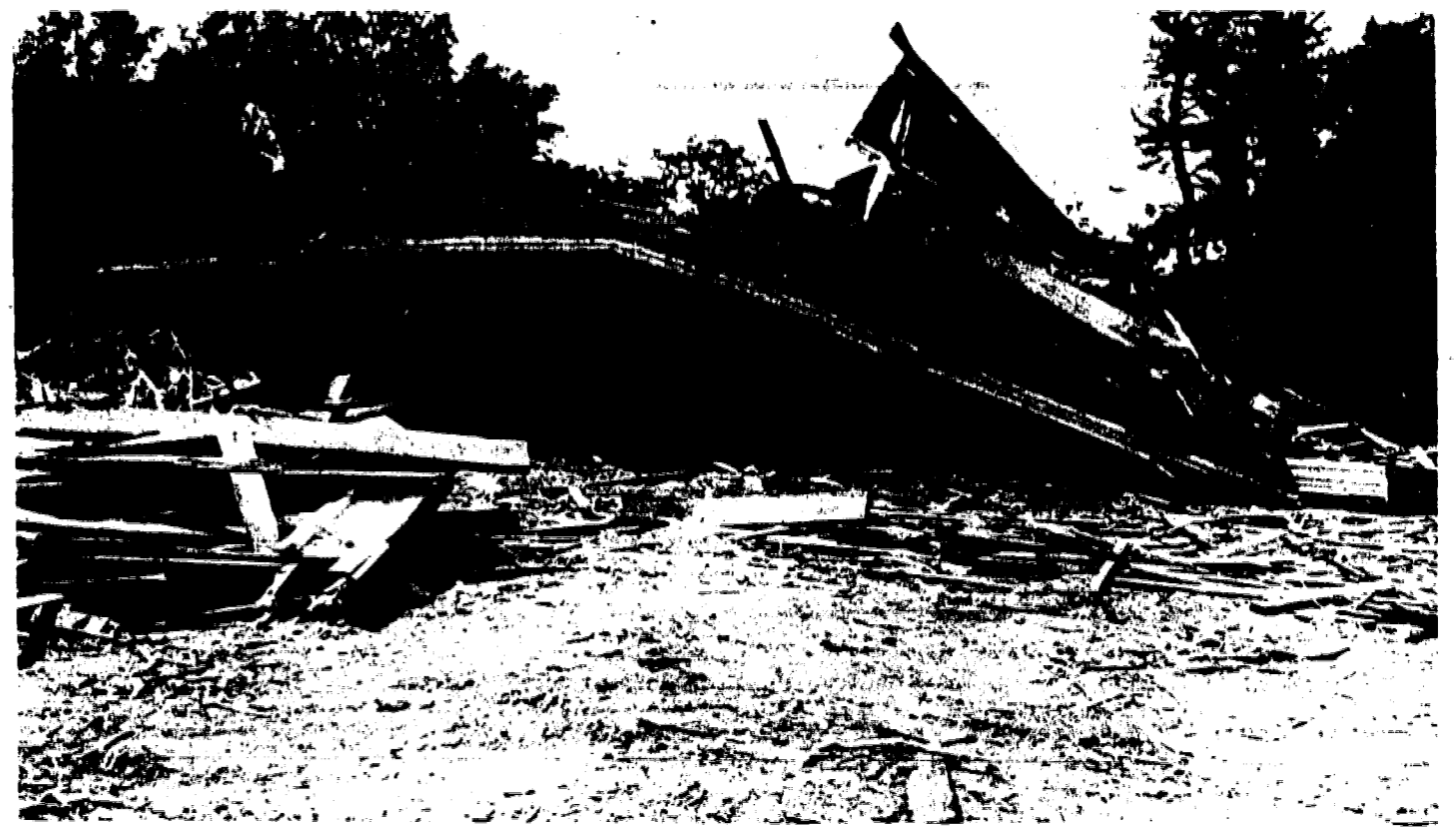
SITE CLEARANCE—A two-story frame building on the Rt. 22 property owned by A.A. Wilson has been demolished but the future of the site is still in doubt. On Monday Wilson asked the Mountainside Board
