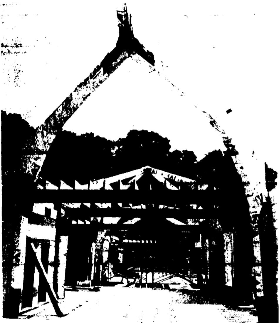
LIBRARY CONSTRUCTION—Steel work is going up for the roof of the new public library under construction on Birch Hill rd. in Mountainside. The one-story building, which will be able to house about 45,000 books, is expected to be completed on schedule by September. (Echo photo by Bob Baxter)
