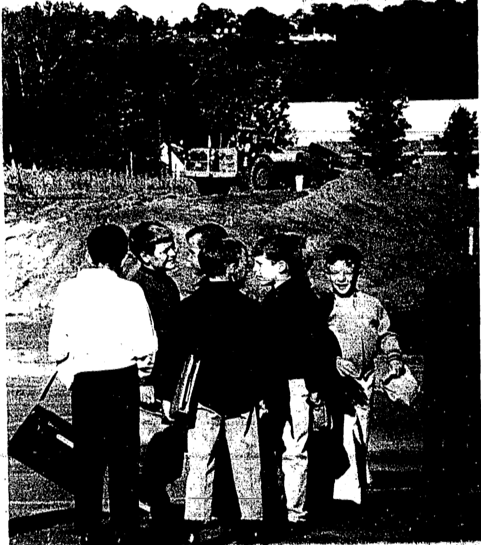
CONSTRUCTION OVERSEERS: Pupils of Deerfield School, Mountainside, do a little "side-walk superintending" of site preparation work for the addition to the school which is scheduled to be ready for the opening of the 1968-69 year. (Echo photo by Bob Baxter)
