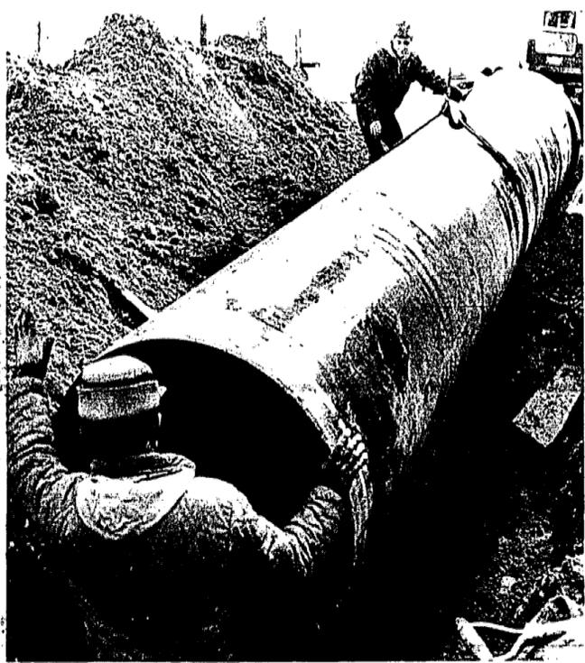
**MORE PIPELINES FOR MORE WATER**—Construction crews put a section of 36 inch water main in place in Mountainside as work progresses on Elizabeth Water's new six-mile pipeline from Scotch Plains to Kenilworth. The transmission main will bring additional water to Hillside and Union and strengthen supplies to Westfield, Mountainside, Kenilworth and Cranford.
