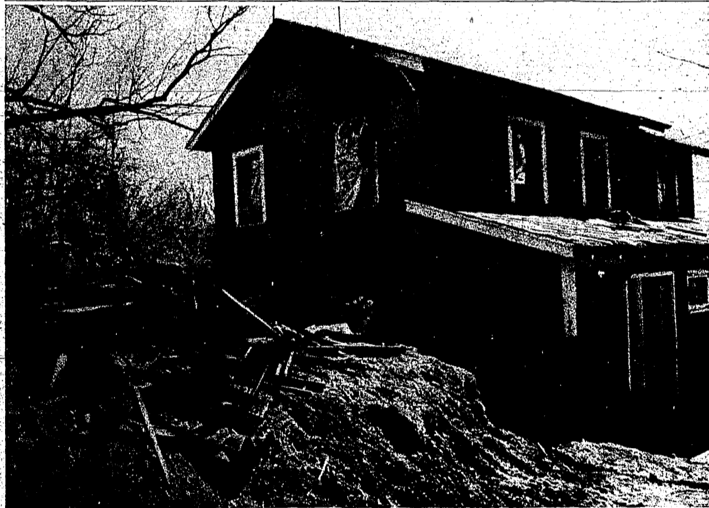
FIRE DAMAGE -- The upstairs of the home of Mr. and Mrs. John Keuler of 161 Locust ave., Mountainside, was gutted last Wednesday night when a fire swept through the upper part of the structure. The Keulers' two children and their three dogs were home when the fire broke out. The children escaped but two of the dogs perished. Mr. and Mrs. Keuler are members of the Mountainside Rescue Squad. She was out on a call and he was attending a meeting at Over-
