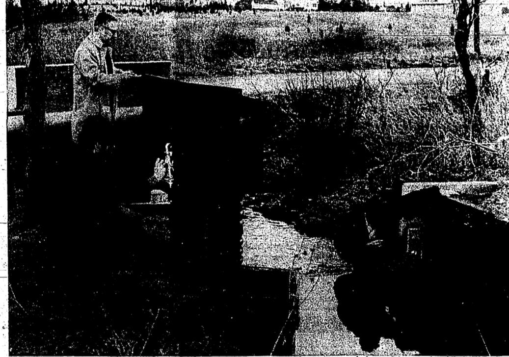
HOW HIGH THE WATER — Rutgers researchers check the calibration accuracy of a stage recorder measuring water depth along a tributary of Royce Brook in Somerset County. George Nieswand (left foreground) examines punched tape of the recorder while Anthony Esser measures water depth with a scale. Kurt Nathan (standing), the project leader, notes findings on a clipboard. They're investigating effects of suburban development on an area's water balance.
