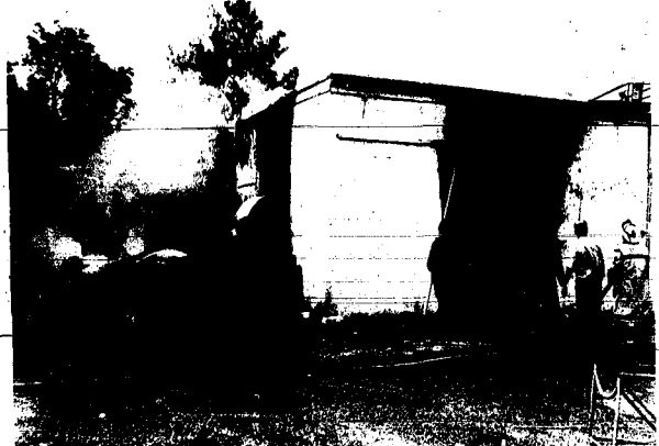
CHECKING FOR DAMAGE — Members of the Springfield Fire Department check the aftermath of a blaze in which a wooden building was completely destroyed and two others were damaged Friday at the Union Free S. C. on Rt. 22. Fire Chief Robert Day said the fire, which was called in at 1:30 p.m., began in the wooden structure where paint was being stored. The blaze then spread to two adjoining buildings where there was minor damage. (Springfield police photo by Howard Thompson)
