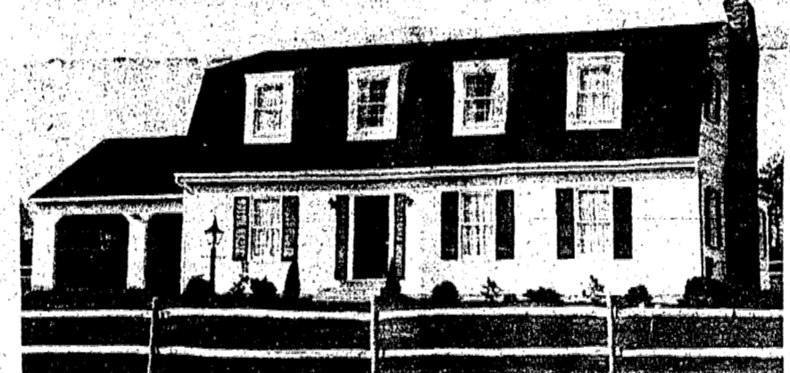
THE SUSSEX—Two fireplaces, four bedrooms and three baths are features of model home in Lawrence Woods, off Cold Soil road in Lawrenceville. For nationally-known builder Carl M. Freeman Associates, this is initial offering in New Jersey—and the four model homes are colonials. Priced at $65,990, the air-conditioned Sussex has sweeping exterior lines and spacious rooms. Home includes two-car garage, full basement, walk-in closets, patio, formal dining room and breakfast room, 20-foot family room, 19-foot living room and two fireplaces.
