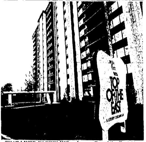
THAT LIVED-IN FEELING — Luxury Top of the East 14-story condominium high-rise is now beginning occupancies on Scenic drive off Route 36 in Highlands. Snyder-Westerlind Corp. of Middletown is developing the 166-unit building which offers one- and two-bedroom condominiums from $38,500. The Applebrook Agency of Middletown handles sales.
