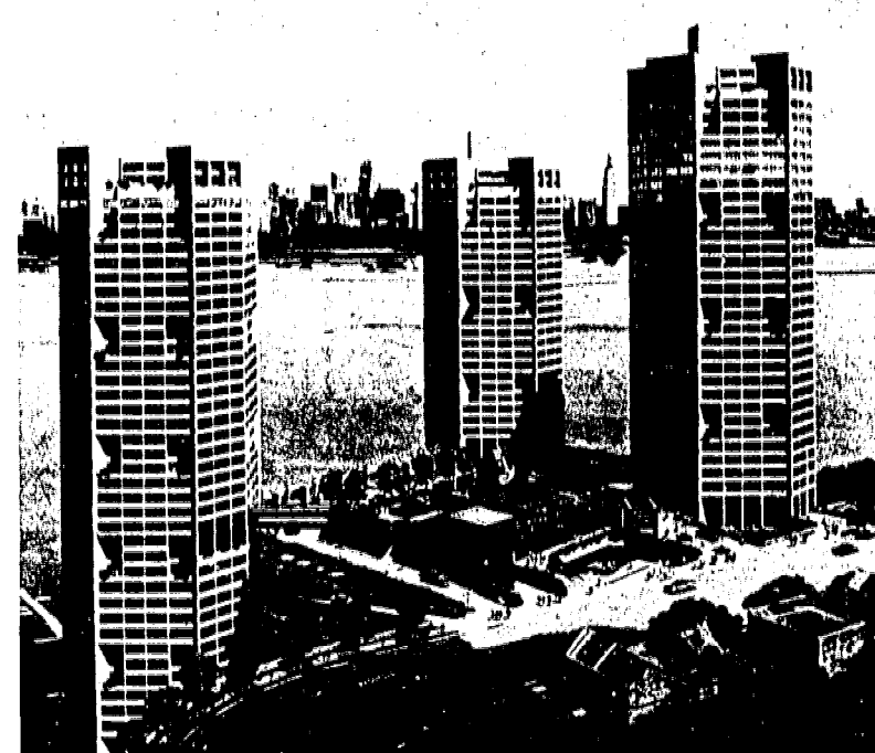
COMMANDING VIEW—Terraces and glass-enclosed solariums will be featured in the 1,200 unit apartment complex, Galaxy, offering residents views of the Hudson River and the Manhattan skyline. In addition to three 43-story residential towers, the five-acre site in Guttenberg will feature recreational and shopping facilities. Opening of the first units and a two-level mall is planned for July.
