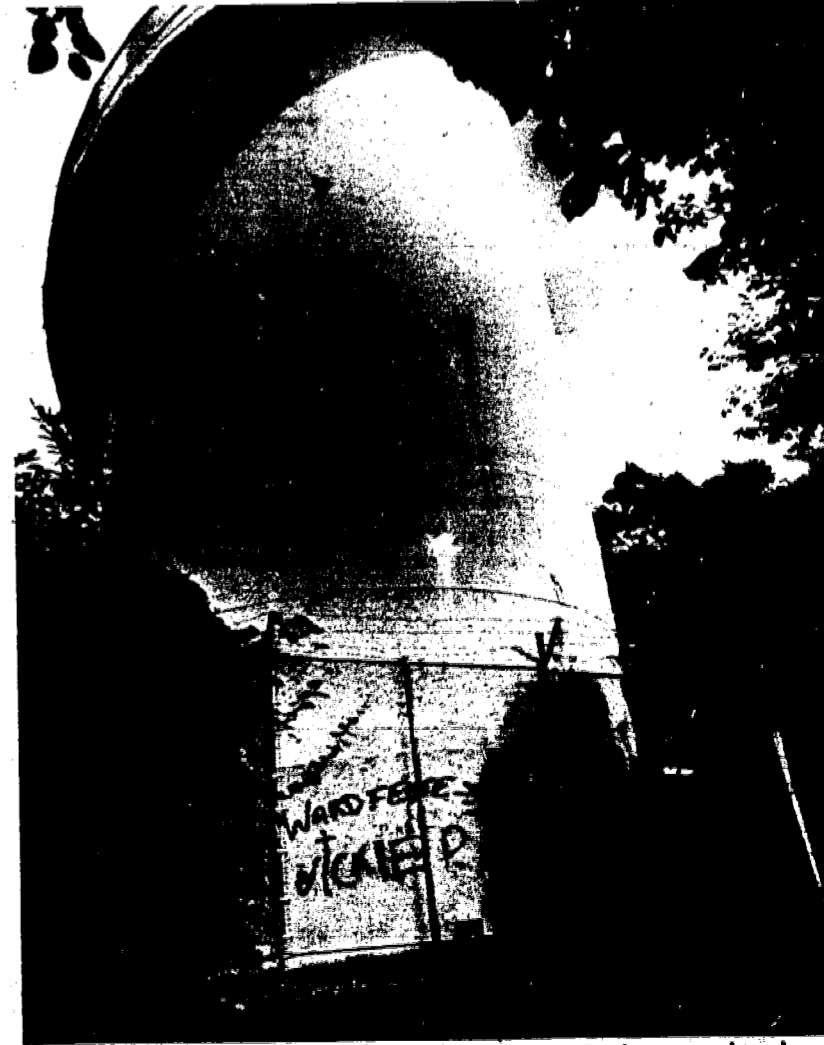
SAFETY PRECAUTIONS —The Elizabethtown Water Co. has completed more than $7,000 worth of safety work on the Watchung Reservation water tower. Officials hope the fencing topped with barbed wire will cut down on accidents and vandalism around the tower. (Glasser Photo Service)
