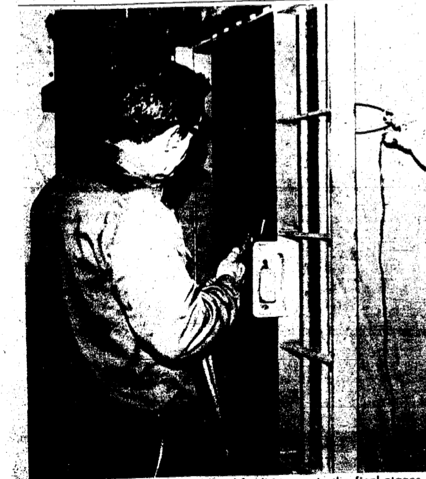
THE LOCK-UP —The new three-cell jail facilities are in the final stages of being installed in the new police headquarters at borough hall. A worker from the Atlantic Coast Jail Co. of Atlantic City welds the lock on the maximum-security cell. (Glasser Photo Service)
