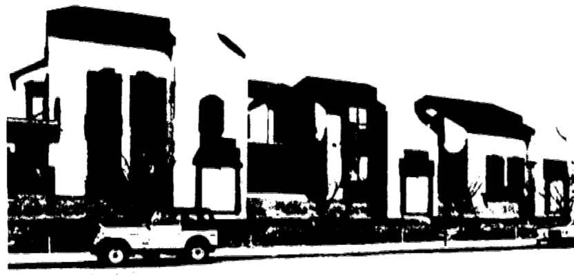
EMERGING SKYLINE —Bayside Villa, a new 25-unit detached patio home community in Perth Amboy, near Smith, High and Rector streets, is in the heart of town which Rosengarten Enterprises is helping to develop. Nineteen different floorplans are offered to buyers who can choose either single-family or two-family models. Prices range from $78,990.
