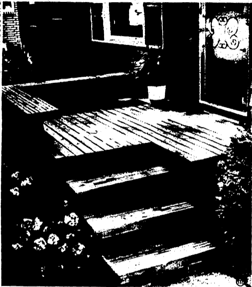
WHAT A WAY TO HIDE — An ugly stoop, that is. This deck is an example of a project you can build to cover a concrete stoop. It's entirely supported by a ledger anchored to the house and by three 4 x 4 posts. The understructure and skirt are made of 2 x 8s; the decking is 2 x 4s. For information on deck projects, send $2 to Georgia Pacific Corporation, The Deck Book, Dept. M, P.O. Box 48406, Atlanta, Ga., 30362.
