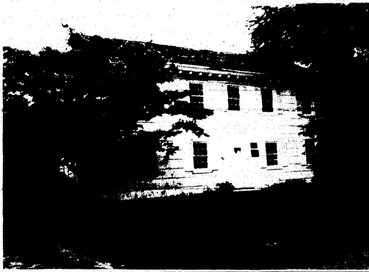
At the Cannonball House, located on Morris Avenue, a barn in the backyard was torn down as part of renovations at the historical site, which is maintained by the Springfield Historical Society.
