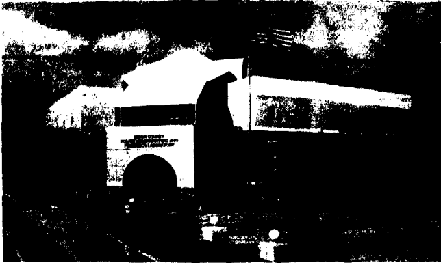
The Musial Group of Mountainside last week presented new plans to the freeholder board for the Union County Police Headquarters in Westfield. Originally, the county had planned to renovate existing buildings on the North Avenue complex but architects have presented another option of constructing a new building.
