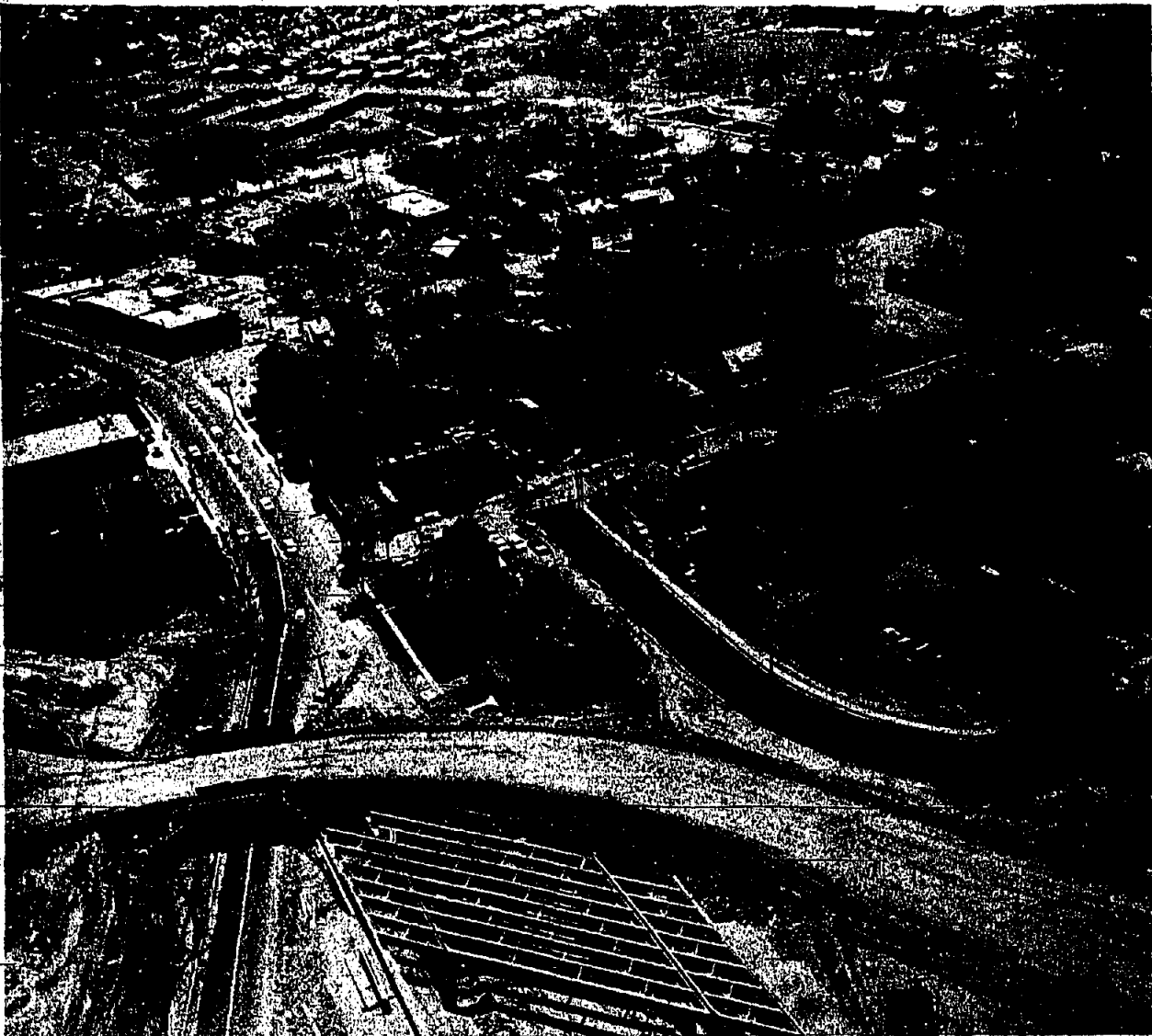
HIGHWAY CONSTRUCTION through the middle of Springfield is clearly indicated by this aerial picture of Rt. 78 as it crosses Morris ave., just west of the main business district. The temporary overpass across a depressed Morris is in the left foreground, next to
