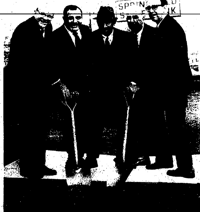
GROUND-BREAKING—At ceremonies Sunday marking ground-breaking for new Springfield State Bank building are (from left) Edward W. Moore, president; Mountside Mayor Thomas Ricciardi, Frank M. Pitt, vice-chairman; Benjamin Romano, chairman, and Springfield Mayor Henry Bulman.
