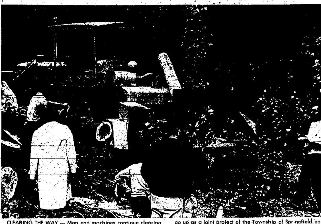
CLEARING THE WAY - Men and machines continue clearing the area between Meisel avenue, Riverside drive and Washington avenue and the Highway Rye, where dikes will go up as a joint project of the Township of Springfield and the Union County Park Commission.
