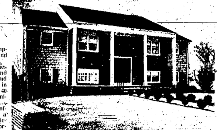
LARGE FAMILY HOMES OF LAGUNA VILLAGE. The quiet residential neighborhood at the front of Laguna Village homes gives little hint of the true waterfront nature of the community, which is located in Point Pleasant. Each of the large family homes (as shown above) backs on one of the wide, deep lagoons that lead out to the waters of Upper Barrington Bay, with easy access to Atlantic fishing grounds. Prices start at $119,000, including home and site spacious...
