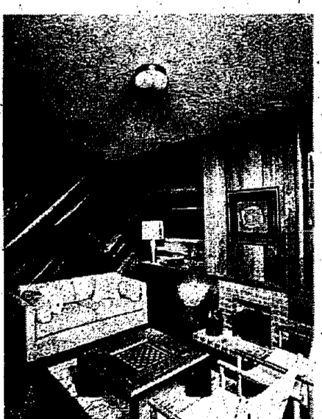
MATCHING IT UP —Accent wall of diagonally applied clear grade redwood lumber in remodeled living room was carefully fit to match horizontal paneling of adjoining wall, adding visual continuity that highlights redwood paneled fireplace. Cabinets were faced with 2/8-inch thick redwood and shelves were installed on movable hardware above (right) for a practical built-in wall unit.
