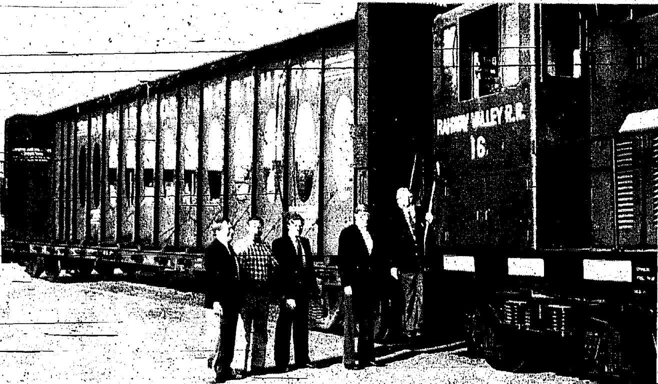
WORKING ON THE RAILROAD —Edward J. Slomkowski, second from right, Union County freemason vice chairman and liaison to the Union County Transportation Advisory Board, joins, from left, William Blust, advisory board representative from Clark; Lowell Jaeger, Jaeger Lumber and Supply Co. owner; Ronald Weching, Transportation Planner for the Union County Division of Transportation Engineering; and Bernard J. Cahill, president of the Rahway Valley Railroad, at the Jaeger Lumber railroad siding in Union. The group met to discuss rail freight service at the firm, one of several industries on the Rahway Valley line that receive and ship raw materials by rail as a direct result of the efforts of the Union County Division of Transportation Engineering and the Transportation Advisory Board to explore ways to maintain essential rail freight services in the county.
