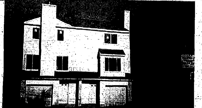
ROSELLE TOWNHOUSES - Pictured is one of the newly constructed townhouses at Amsterdam Place in Roselle.
