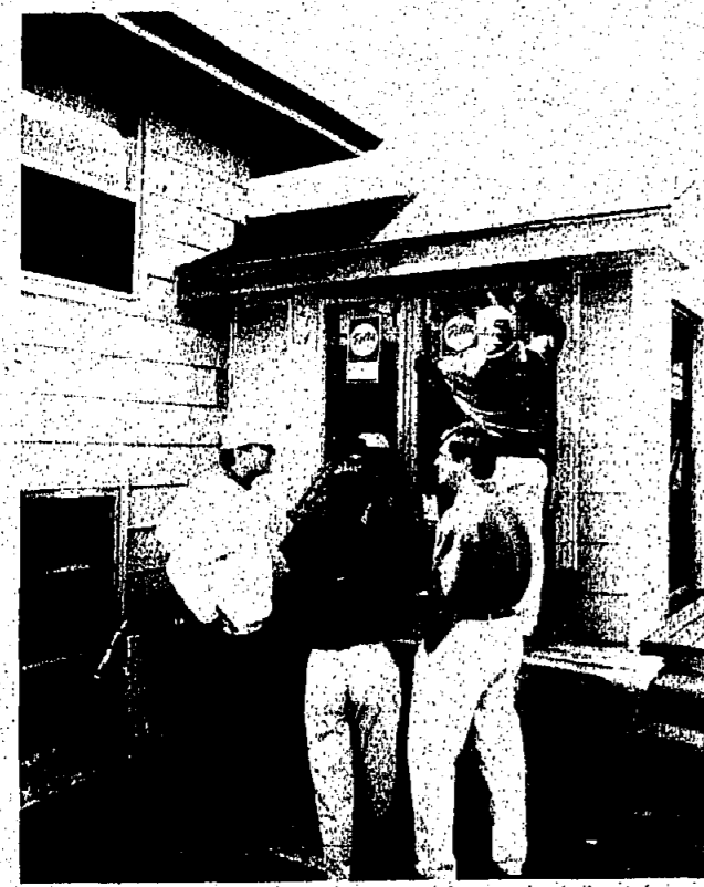
Workers from Pella Windows and Doors install a window on a remodeled home.
