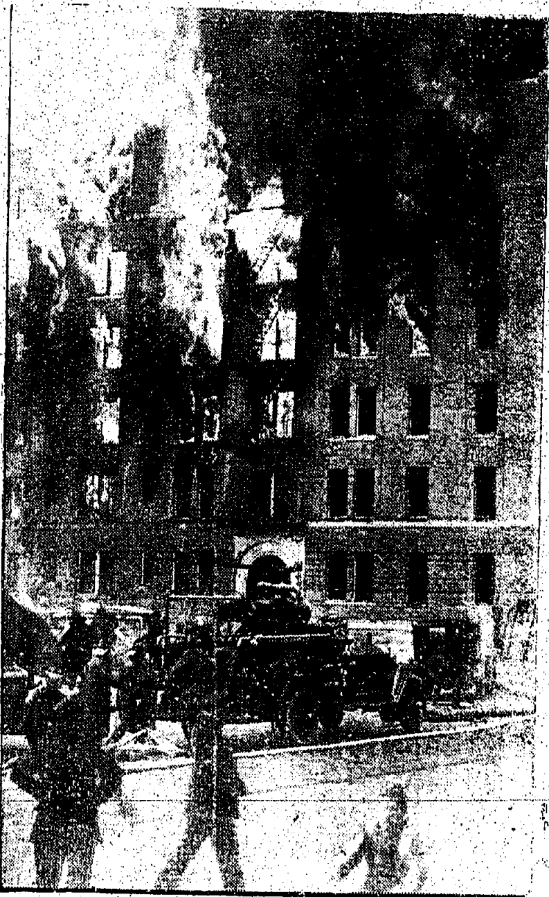
FLAMING THREAT against arson probe. This spectacular fire, occurring in unfinished six-story apartment house in New York city, has been linked with investigation of arson ring operating in upper New York. Building is owned by corporation of which Henry O. Heuer, a member of grand jury probing suspicious fires, is secretary. An infernal machine is thought to have been used in starting fire, which cost one life.
