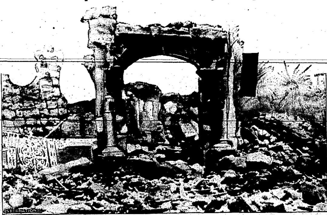
Ruins caused at Managua by the most disastrous earthquake in the history of the country. More than 2,000 persons lost their lives.
