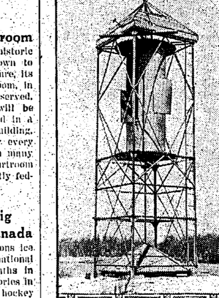
On the estate of Charles L. Lawrence at East Islip, L. I., may be seen the rotor windmill in operation in this country.
