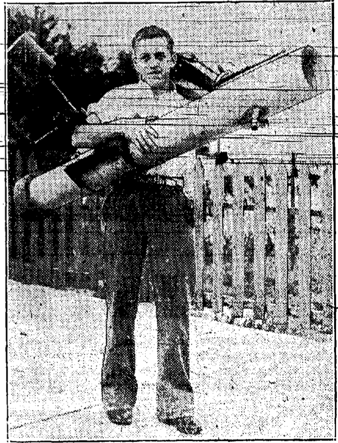
STUDENT CONSTRUCTS PORTABLE TELESCOPE —Arnold Oswald, Los Angeles Junior College student, carrying his 30-pound portable telescope, which he constructed in his spare time at a total cost of $30. Made of parts of various instruments in his home, it is an accurate 6-inch reflector type and magnifies to 160 diameters.
