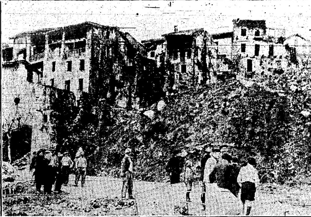
FRENCH TOWN WRECKED BY LANDSLIDE —A view of some of the ruined homes in Roquebillieres, near Nice, after the town had been half buried by a heavy landslide caused by torrential rains.
