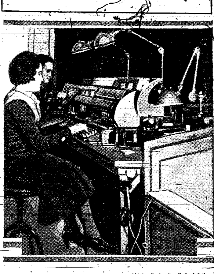
Photograph, Canadian National Railway. THAT the ticker tape machine shown in the photograph is capable of recording 500 characters per minute. It is the latest device installed by the Canadian National Telephone to report stock exchange transactions and in one trading day it can handle 1038 feet of ticker tape and record 150,000 characters. The maximum recording speed of the machine in use before this one was 150 characters per minute. The machine is operated on the typewriter key board principle.
