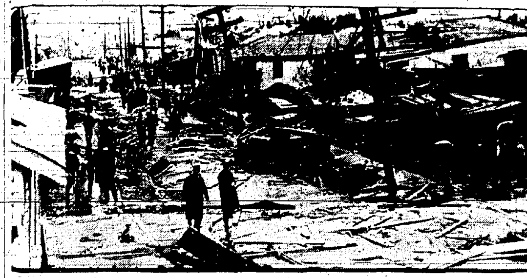
A general view looking down Ends street, New Orleans, showing the damage wrought by a wind storm. One hundred homes were demolished.
