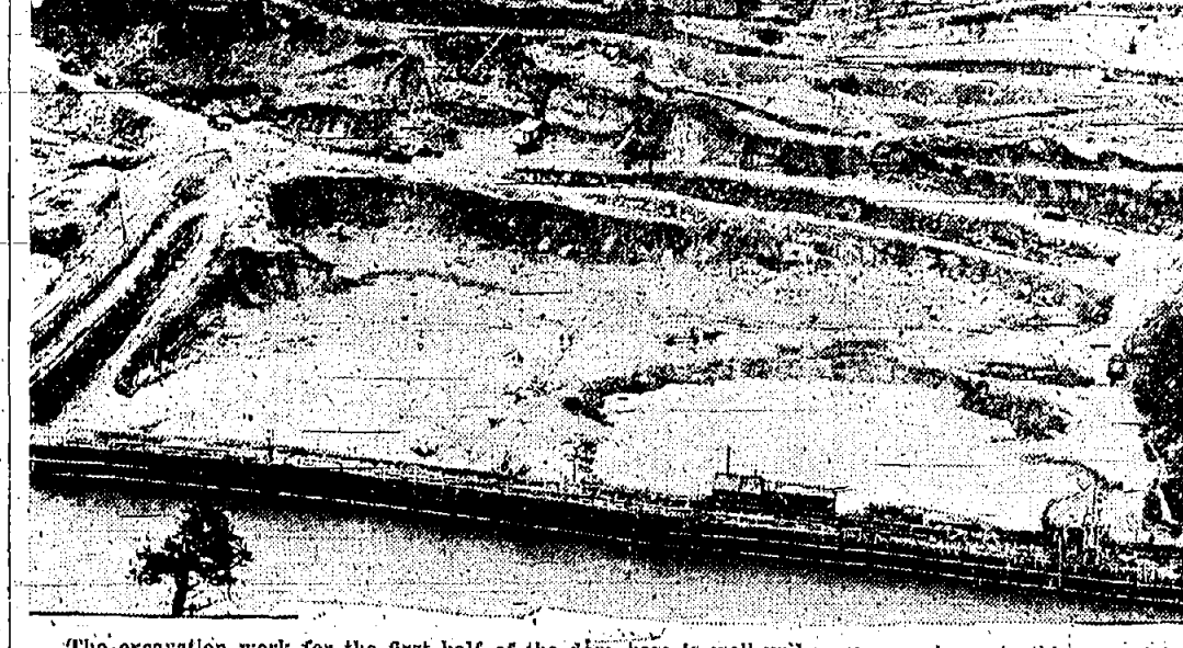
The excavation work for the first half of the dam base is well under way, as shown in this new picture of the Norris Dam project in Knoxville. The excavation work extends about fifteen feet below the river bed, and digging will be continued until solid rock is reached.
