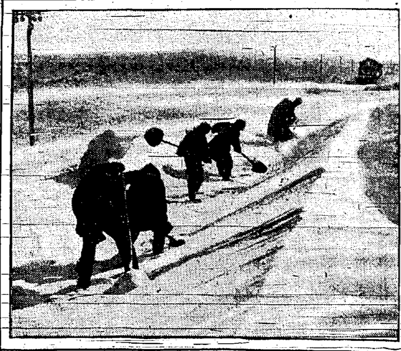
Clearing the tracks of a railroad in the Sahara clogged by shifting sand dunes as the train waits in the distance.
