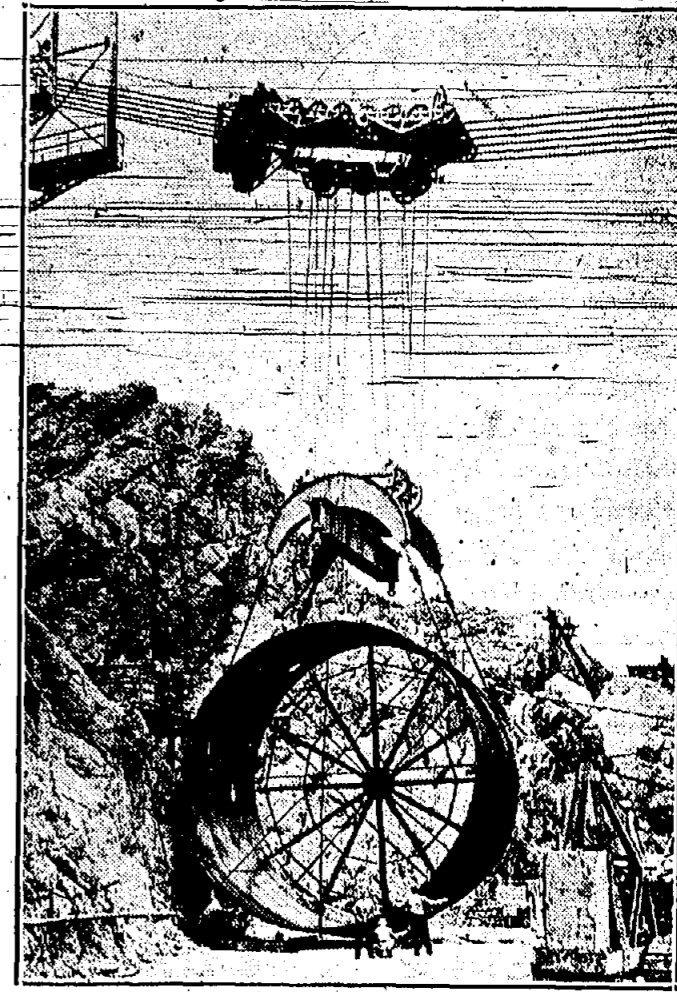
90-TON PIPE SECTION FOR BOULDER DAM —The largest section of steel pipe ever fabricated for an engineering project was recently placed in final position in the upper Nevada intake tower of the great Boulder Dam project. Here is the pipe being moved. Weighing 90 tons, it is 30 feet in diameter and 21 feet long.
