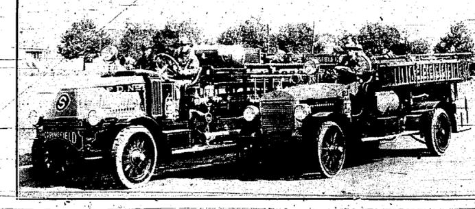
The two largest apparatus of the Springfield Volunteer Fire Department, the Mack hose wagon and chemical truck on the right and the hook and ladder combination hose pumper and chemical truck. Both vehicles have been in service since 1925.
