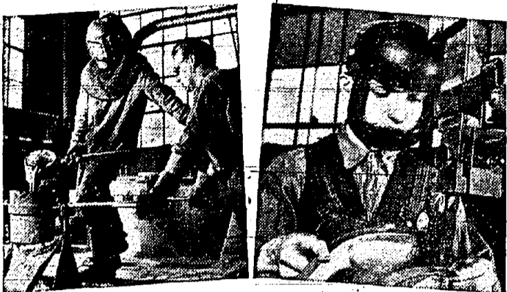
Wearing heavy, metal shoes, a freeproof suit and a helmet that looks like a diver's, a worker pours molten metal.
