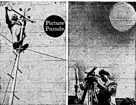
HIGHBOY . . . The gentleman atop the pole is adjusting the cup anemometer and wind vane, a device for determining the speed of the wind.
