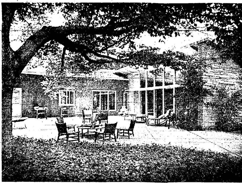
REAR VIEW of "luxury home," Seven Oaks Park, Orange which was opened to the public last Monday.
