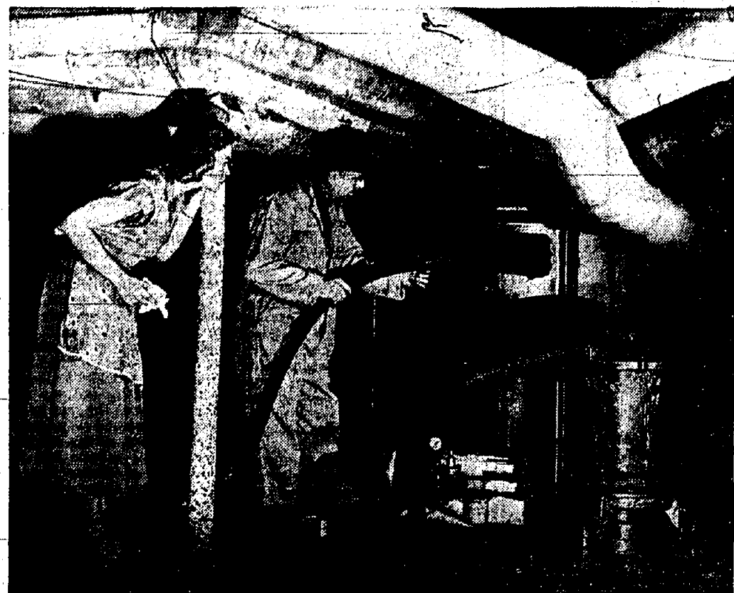
DON'T FORGET the furnace. Be sure to have it cleaned out by an experienced repairman. Chimneys, the flues and smokepipes should also be inspected, for cracks through which the heat may escape.
