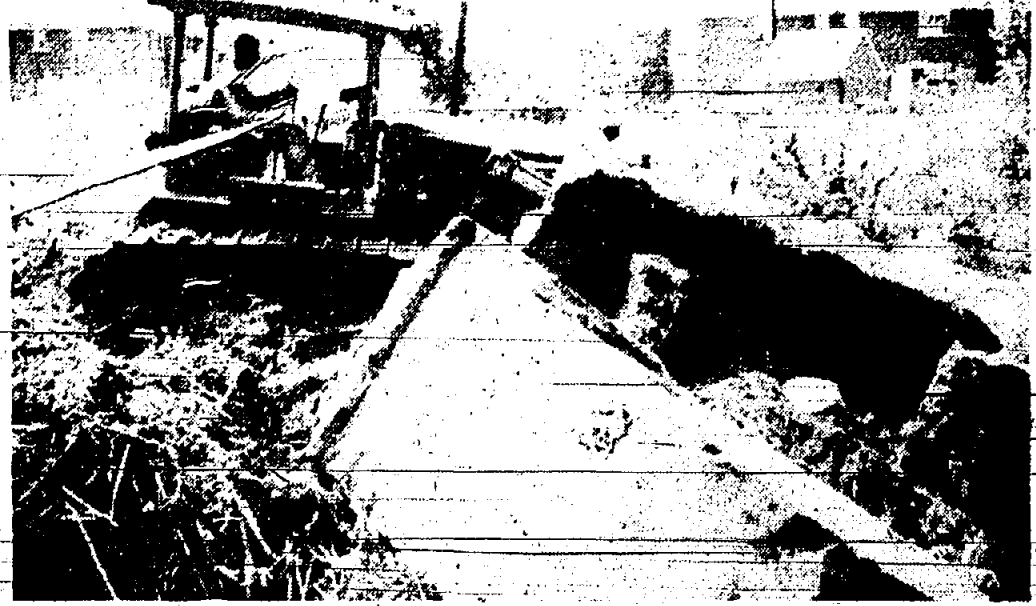
CLEARING THE WAY —Construction of dozer cleared the area of trees, old building foundations and debris and paved the way closer to reality as the above-pictured bulldozer gets started on the actual construction work.
