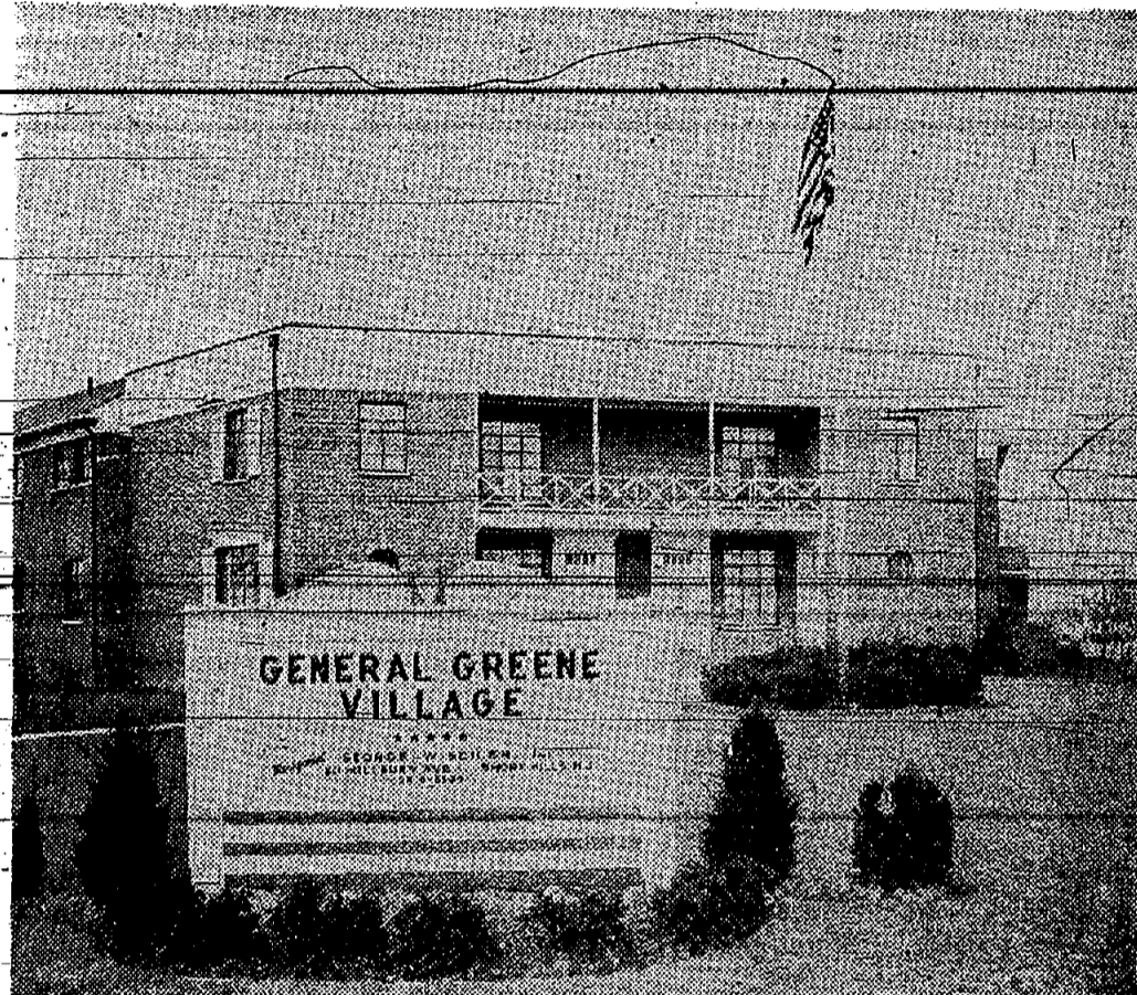
PART OF FIX UP WEEK. General Greene Village has that "new look" since William J. Chirgottis took over ownership of the apartments here in Springfield. Photo shows new landscaping and flag pole to conform with "the fly more flags campaign" being urged by the Lions Club. The beautifying project has been extended to all part of the apartment village. (Photo by Mickey Fox)
