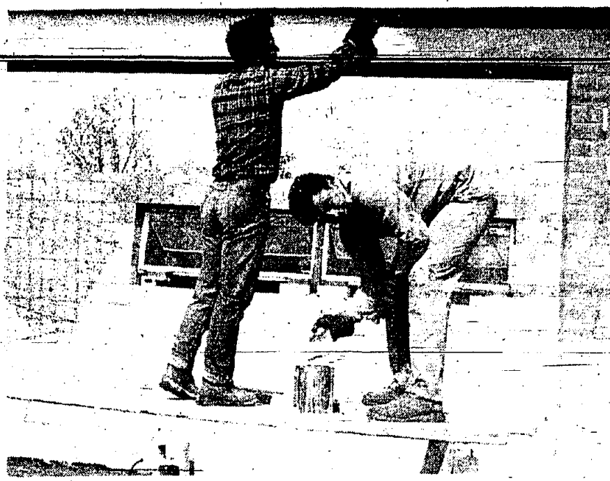
WORKMEN PAINT THE GIRDERS on the new bath house at the Municipal swimming pool. Progress on the pool construction is moving along smoothly. The pool should be ready for use early this summer.
