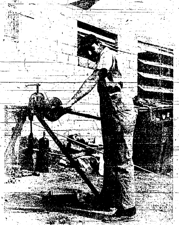
APRIL 29 - WORKMAN HASTENS TO COMPLETE PLUMBING INSTALLATION.
