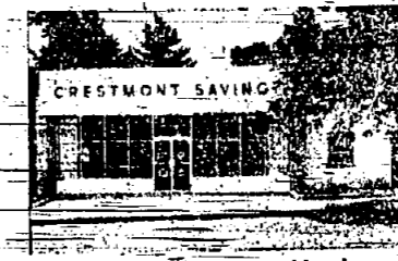
1040 Chancellor Ave., Maplewood
