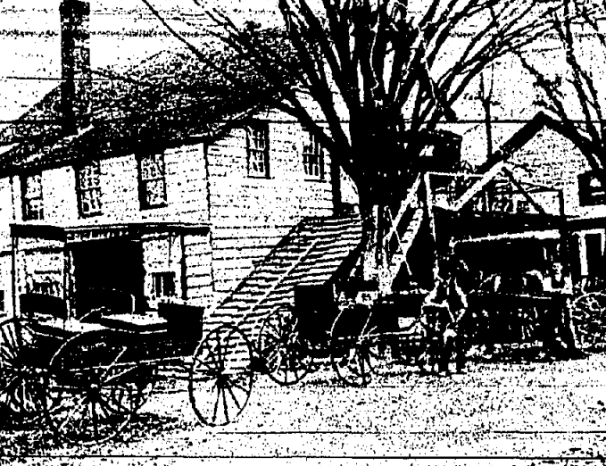
Farrow's Carriage Shop on Springfield Ave., where the body shop of Dobbs & Co. is, is not, as it looked in 1897. The ramp was used to haul carriages to the second floor for painting.
