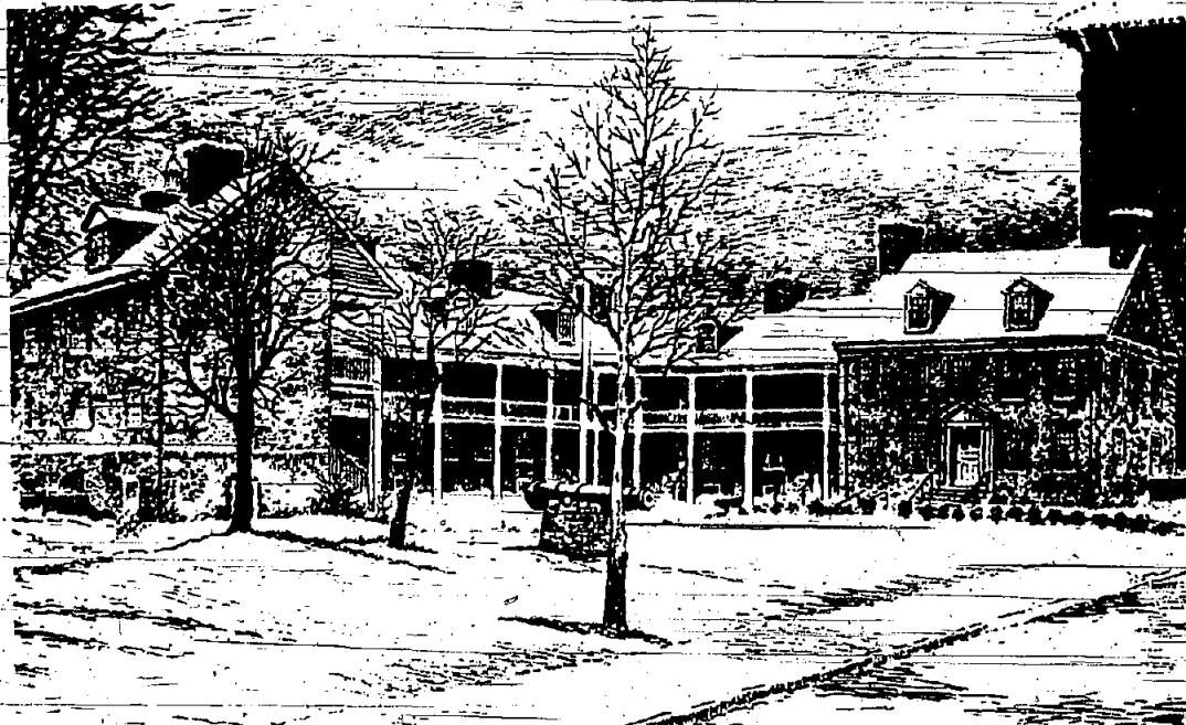
RESTORED OLD BARRACKS in Trenton, from etching by G. A. Bradshaw. This is only one of five original barracks still in existence in New Jersey.
