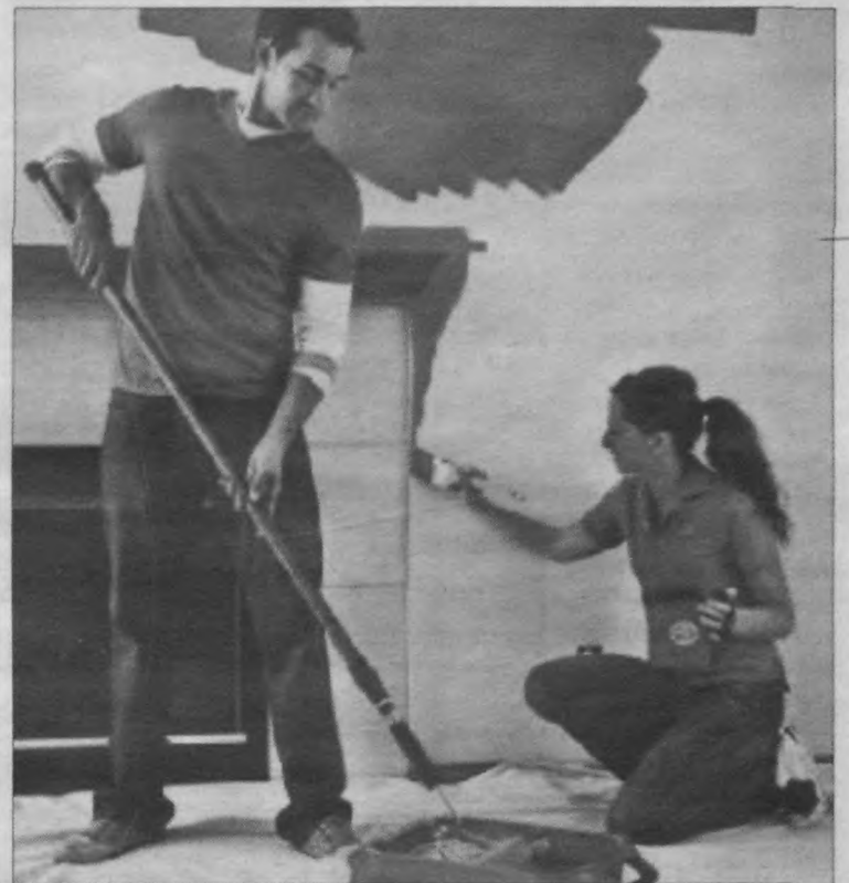
Painters can reduce the stress of a mess by protecting floors with old bed sheets or canvas, and covering woodwork, glass and metal surfaces with painter's tape.
