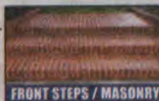
FRONT STEPS / MASONRY
