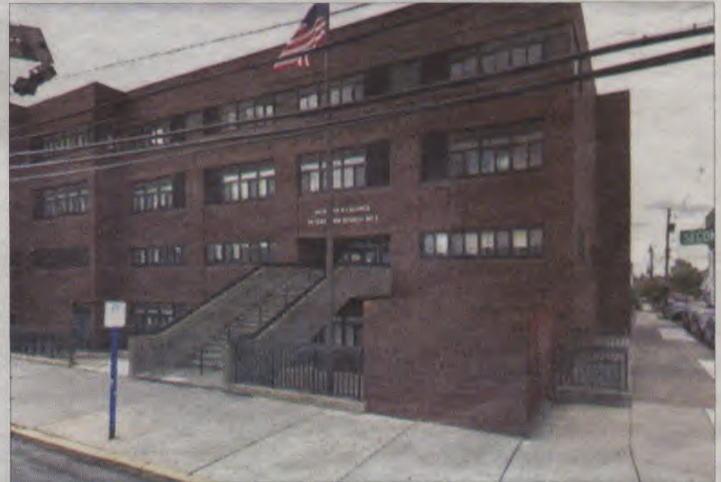
Photo Courtesy of Google Maps
